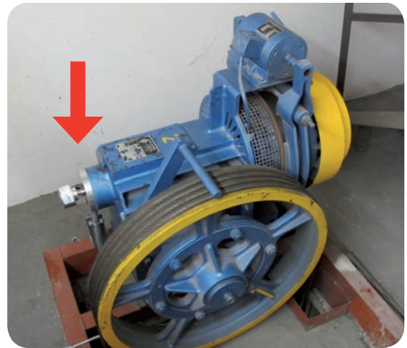
Example: KASPER drive KP120 with encoder mounting
