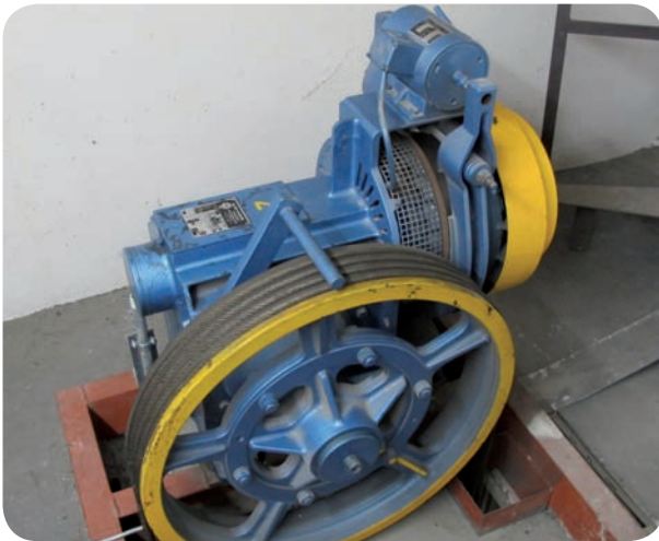
Example: KASPER drive KP120 without encoder mounting
