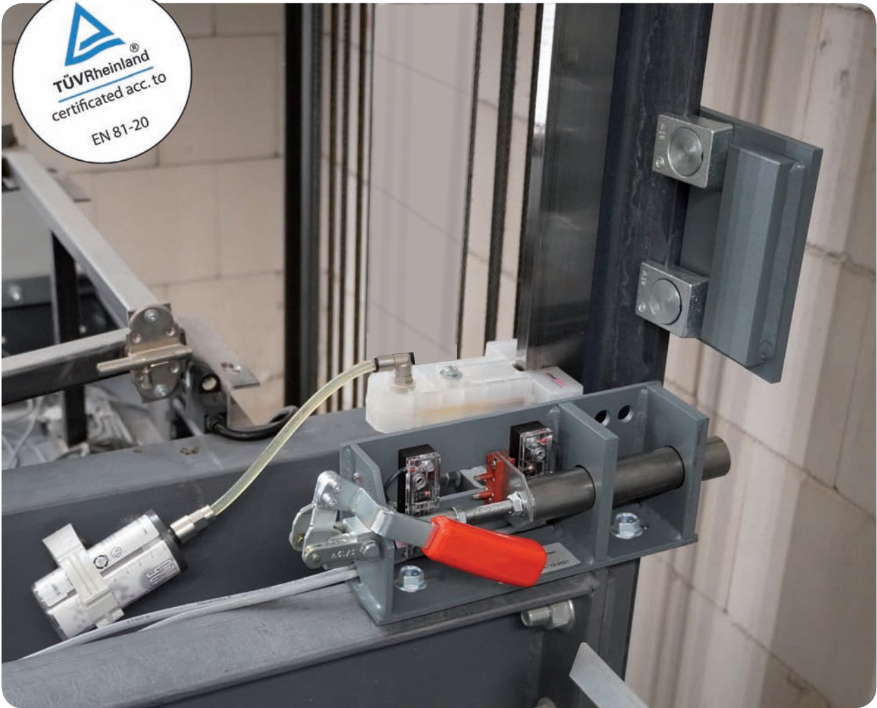
Mounting example travel path limitation
